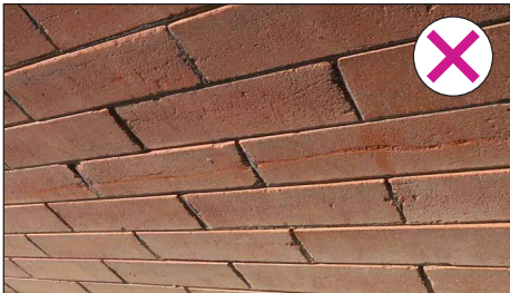
Repoint missing or deteriorated joints with an appropriate, compatible mortar | Post Oak Preservation Solutions
