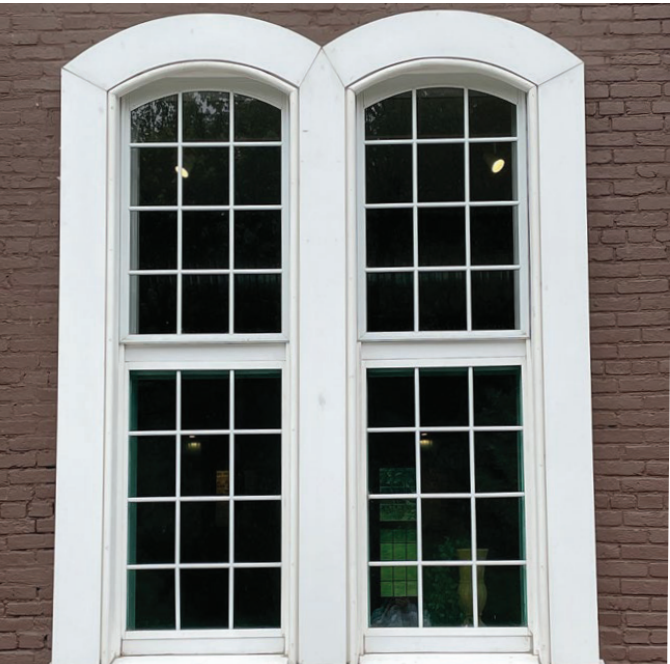
Figure 9. Previously bricked-in openings below the flood line were reopened and new aluminum windows installed with cellular PVC trim detailed to hold back moderate flood waters and survive exposure to water. Photo: John Sandor, NPS.
