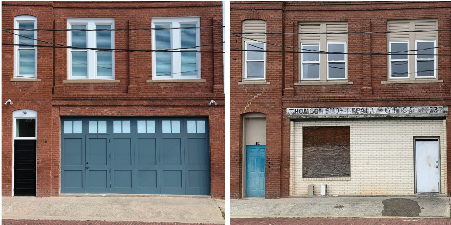
Figure 20. Cement board was used to replace a non-historic infill and mimics the configuration of a typical vehicular door of the period. Photos: Historic Augusta.
