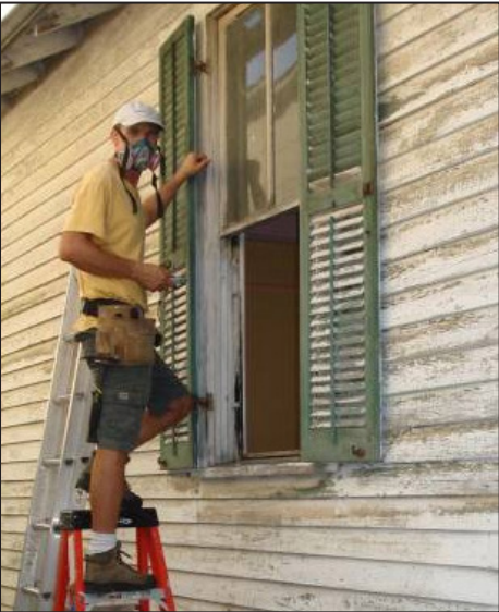
Maintain existing paint coatings on exterior wood to prevent exposure to wind, sun, and rain | Post Oak Preservation Solutions
