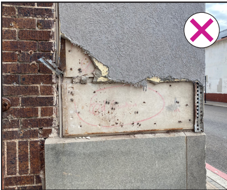
Covering historic masonry can cause damage to the underlying historic material | Post Oak Preservation Solutions
