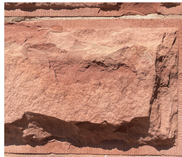
Figure 13. Cast stone was used to effectively replace individual blocks of sandstone. Both the original (left) and the substitute material (right) retain similar physical and visible properties. Having weathered for over 30 years, some erosion of the binder has revealed quartz grains of the aggregate (inset), but it is only noticeable upon close inspection. Photo: John Sandor, NPS.
