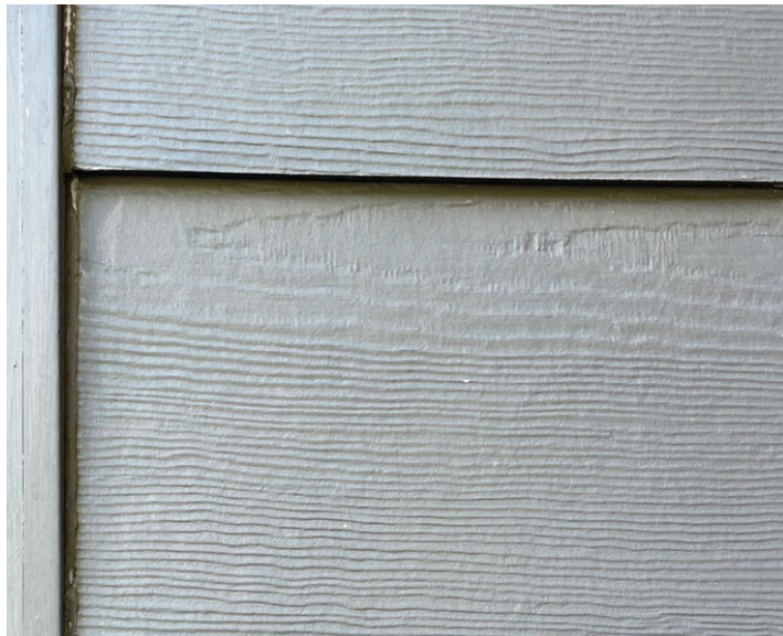
Figure 14. Surface texture is an important aspect in matching the appearance of a historic material, especially when a material is viewed at close range. As seen in these two images, many of the substitute materials produced for siding and trim have an embossed wood grain, making them incompatible for replacing historic wood that was typically planed to a smooth surface. Some substitute products are available with a smooth surface as well. Photos: John Sandor, NPS.
