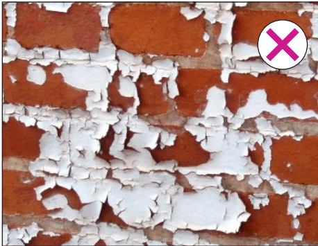
Non-historic paint coatings and water repellent treatments are inappropriate for historic masonry | Post Oak Preservation Solutions
