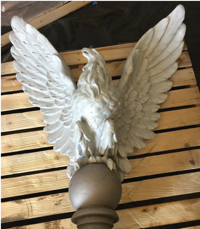
Figure 16. Aluminum is a highly corrosion-resistant metal that is commonly used as a substitute material for cast iron. Aluminum can be a more affordable and lightweight alternative to cast iron that retains a similar texture, shape, and maintenance cycle. Photo: NPS.
