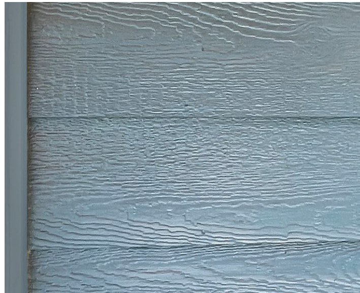
Figure 14. Surface texture is an important aspect in matching the appearance of a historic material, especially when a material is viewed at close range. As seen in these two images, many of the substitute materials produced for siding and trim have an embossed wood grain, making them incompatible for replacing historic wood that was typically planed to a smooth surface. Some substitute products are available with a smooth surface as well. Photos: John Sandor, NPS.
