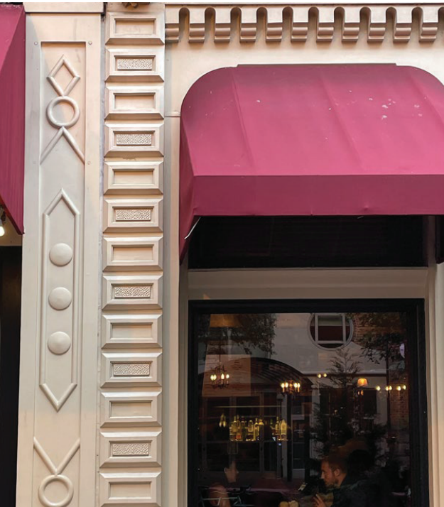
Figure 2b: The 19th century also produced a variety of metal products used to imitate other materials. Across the country, cast iron was used in storefronts to imitate stone. Photo: John Sandor, NPS.
