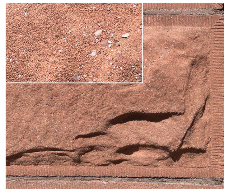
Figure 13. Cast stone was used to effectively replace individual blocks of sandstone. Both the original (left) and the substitute material (right) retain similar physical and visible properties. Having weathered for over 30 years, some erosion of the binder has revealed quartz grains of the aggregate (inset), but it is only noticeable upon close inspection. Photo: John Sandor, NPS.
