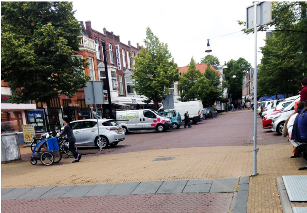
Figure 4.18 | Raised intersections and crosswalks support walkability and pedestrian safety | Northeastern Delft CC 2.0
