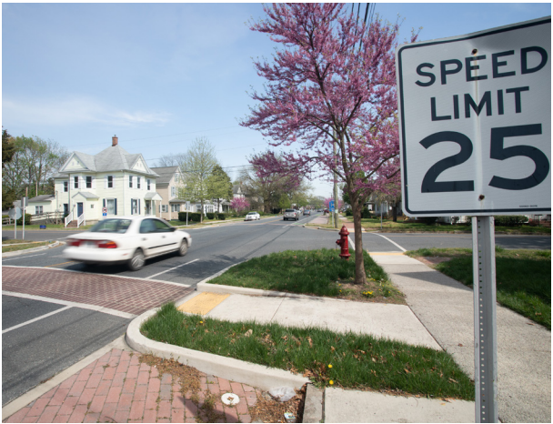
Figure 4.8 | Bulb-outs reduce runoff and slow traffic | CBP CC 2.0
