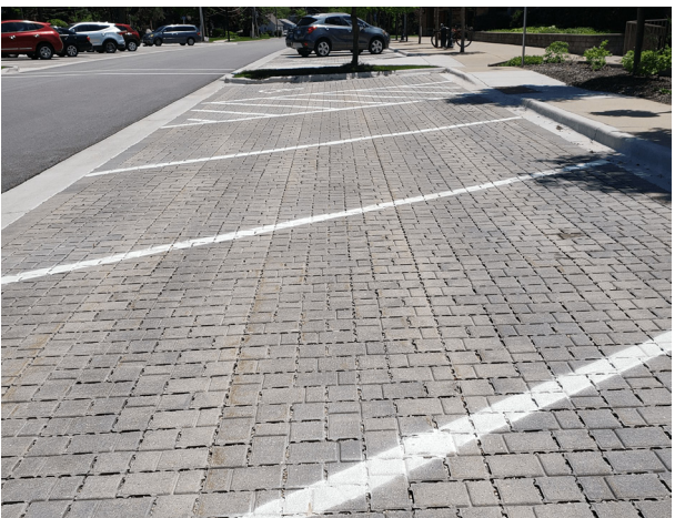
Figure 4.10 | Permeable pavers reduce storm runoff | City of Warrenville
