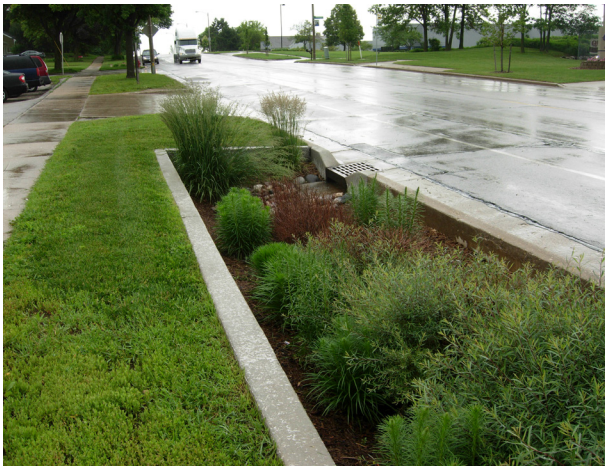
Figure 4.9 | Biofiltration reduces and cleans runoff | A. Volkening CC 2.0
