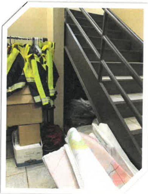
Under stairs storage
