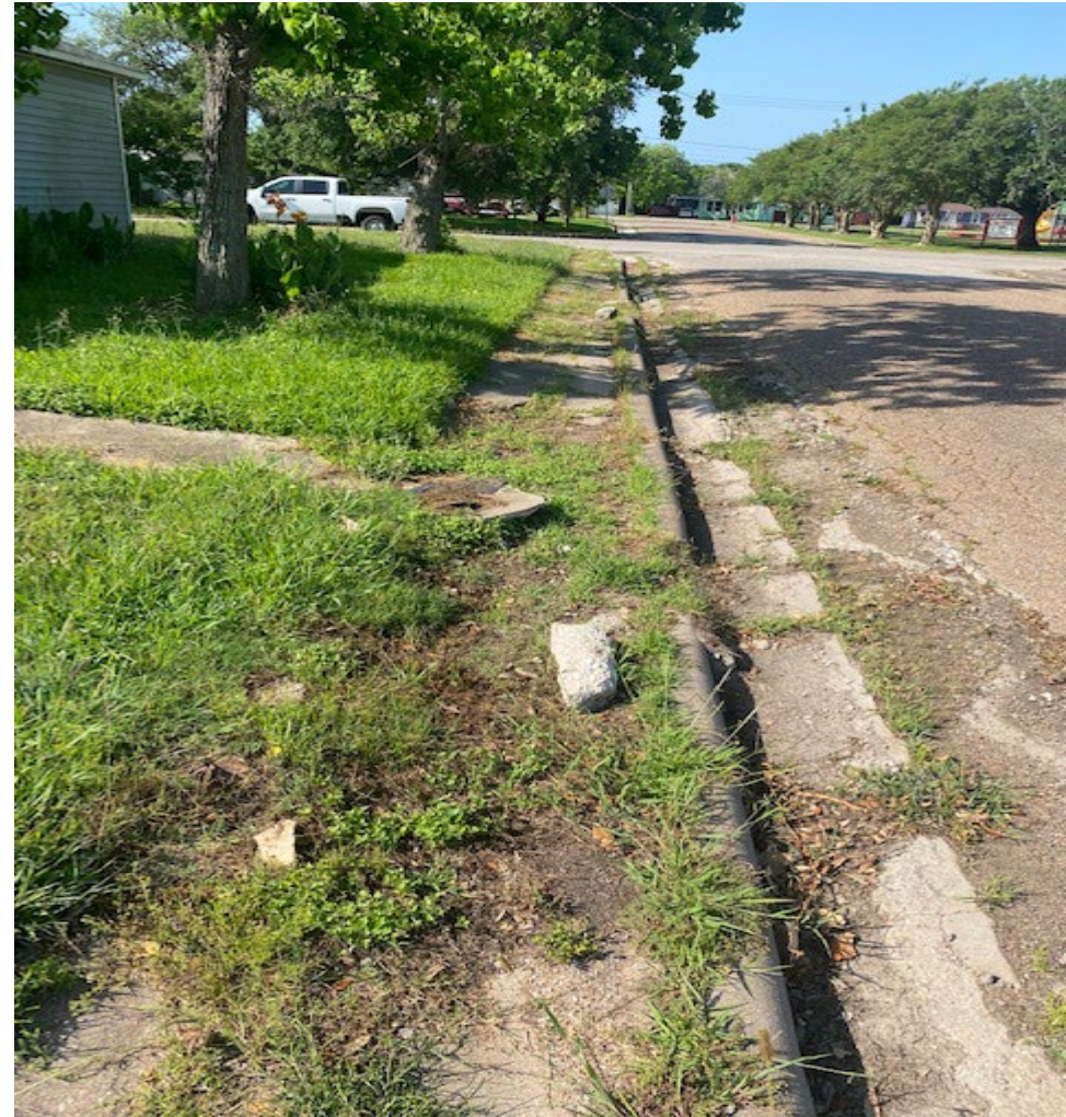
1130 8 th Street to Alley
