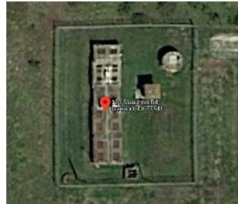
Slaughter Road Treatment Plant Wastewater Treatment Plant (Slaughter Road WWTP)
