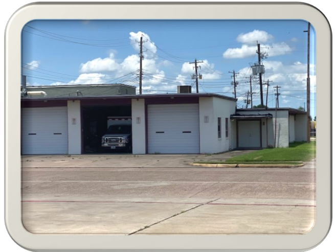
Old Fire Station 128 East Fourth St.
