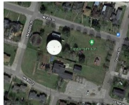
8 th St. Booster Pump Station
