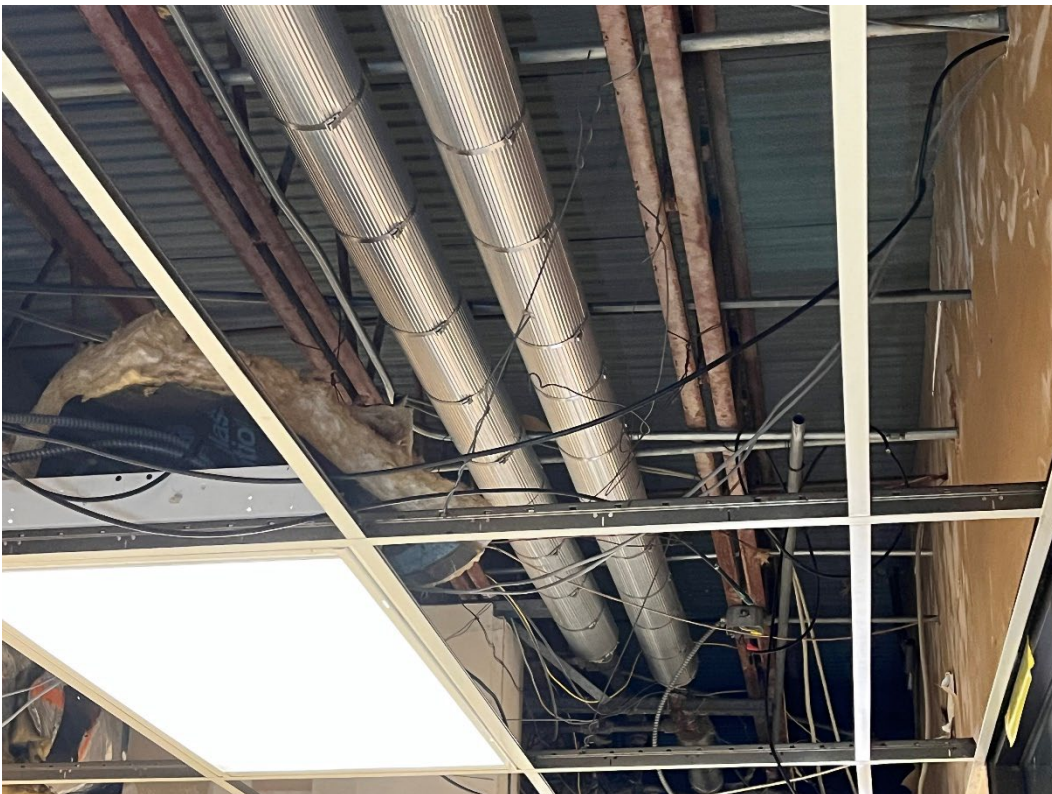
Photo #26: View of piping in hallway – Level 2 – Corridor 223.
