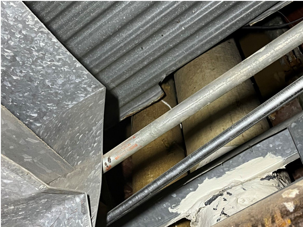
Photo #6: View of vertical pipe chase above first floor ceiling.
