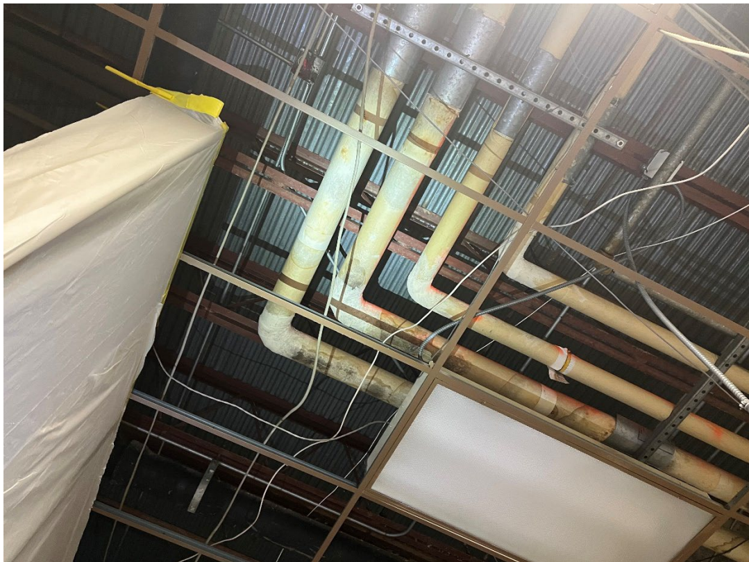
Photo #10: View of the pipe fittings – Level 1 - northeast room 125.
