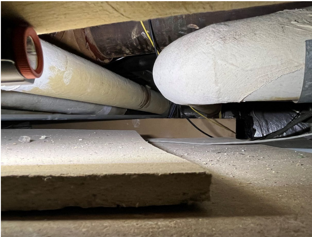
Photo #8: View of pipe fittings above Level 1 ceiling – Room 117.
