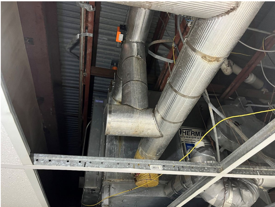
Photo #24: View of piping on air handler – Level 2 men’s restroom.
