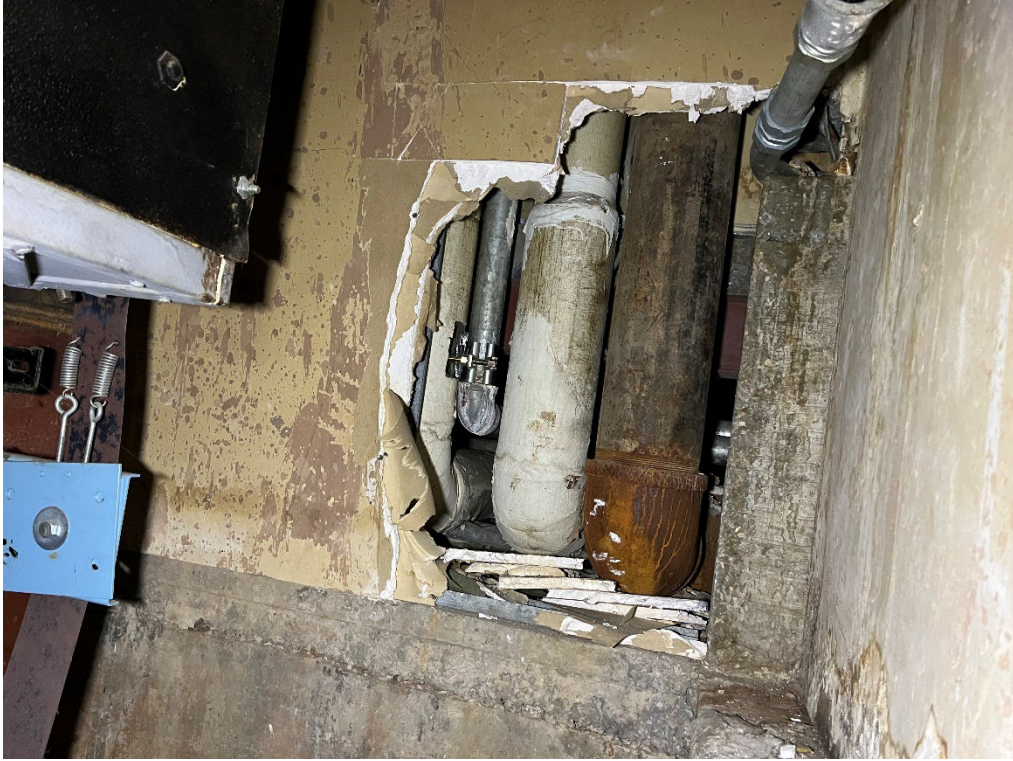
Photo #5: View of pipe chase – north side of elevators.
