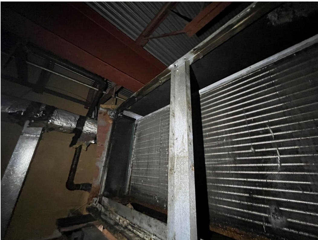
Photo #28: View of evaporator coil and framing – above southeast restroom.
